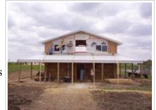
Submitted The Sustainable Living Coalition built this 1,200-square-foot straw-bale, post-and-beam barn as a main classroom and administrative space.
