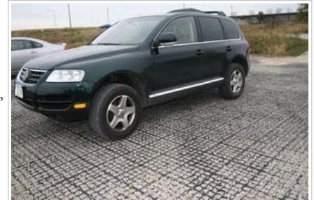
Ann Scholl Rinehart This parking lot at the Urban Steward Alliance Rain Water Management Project site in Fairfield, Iowa, is an example of eco paving.
